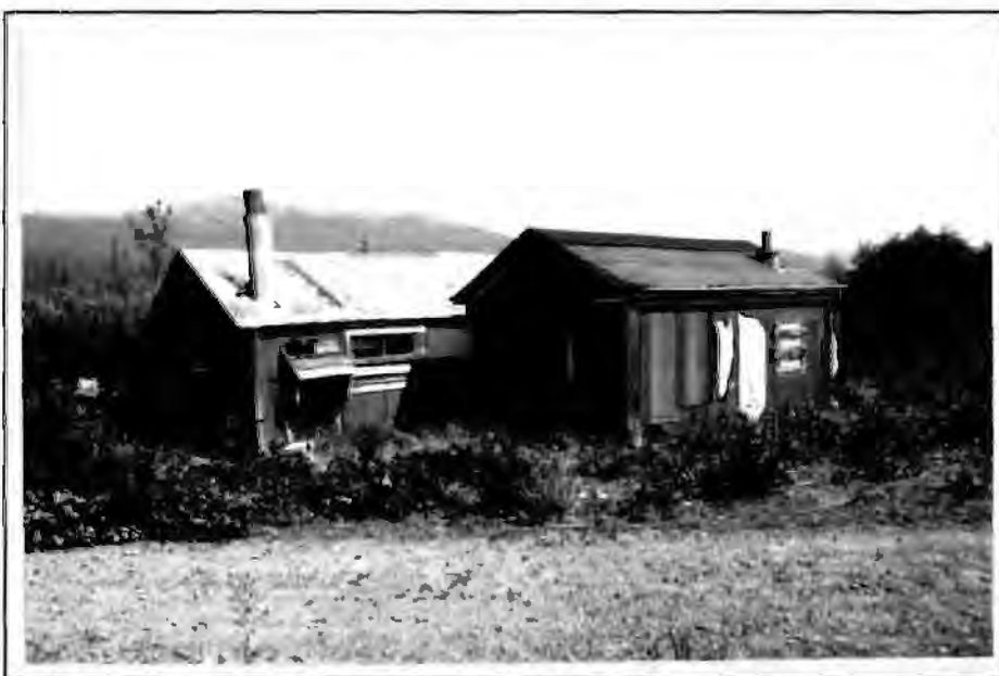
Figure 55. The Matheson Mess Hall (left) and Cook's Quarters (right), 1993. The view is looking northeast.
